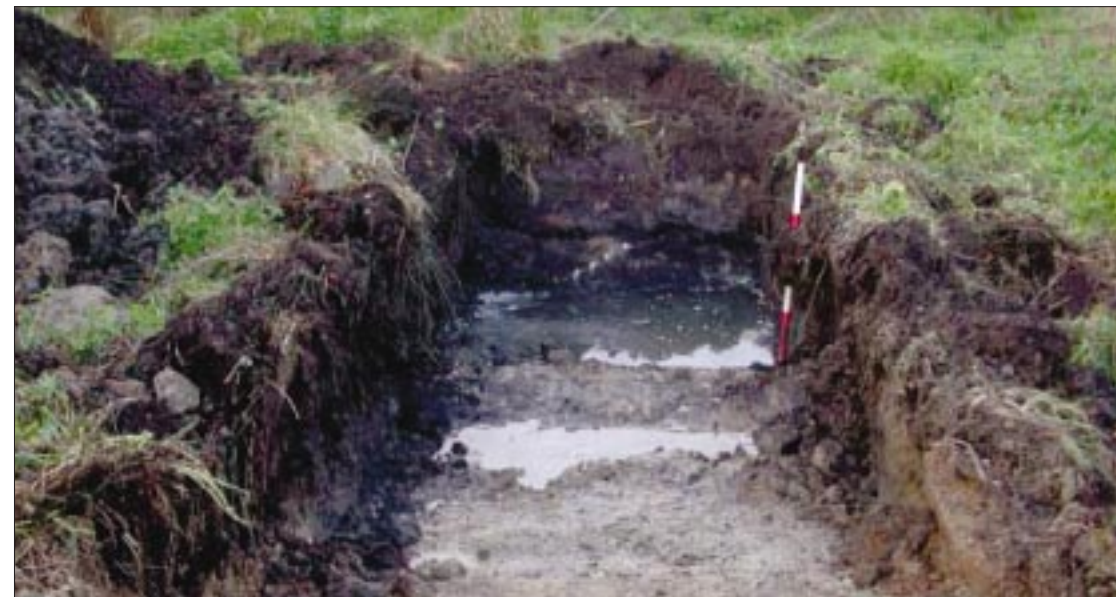
Plate 7 Trench 5 - Western end of trench with large cut filled with water, section showing backfilled with modern dump
