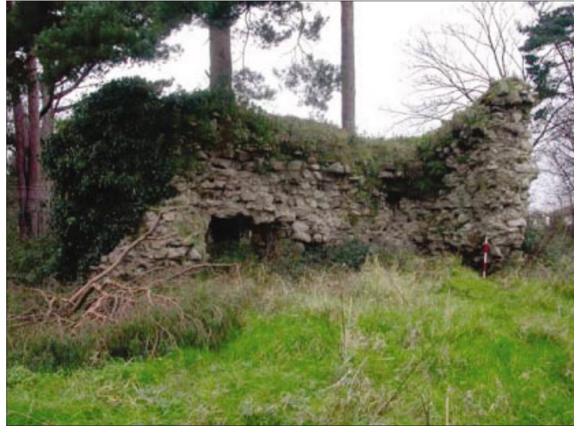
Plate 2 Current state of Murphystown Castle remains from the north
